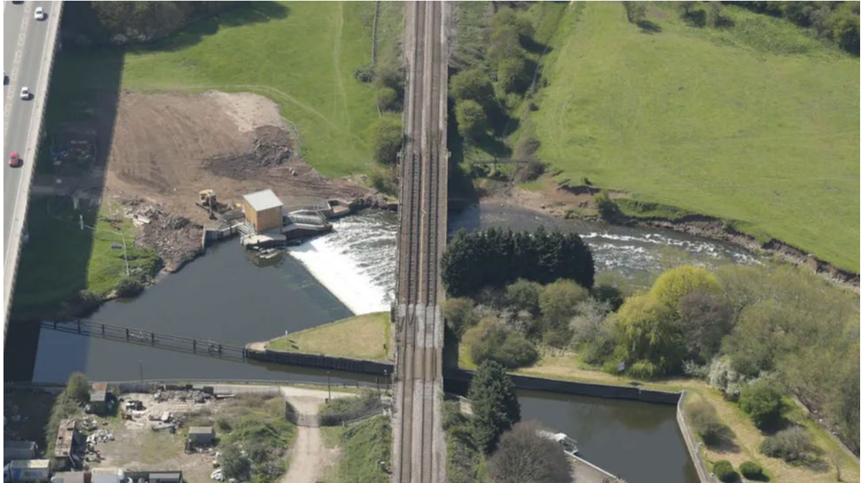
River Devon Trent showing the weir and Hydro-Electric Power station
